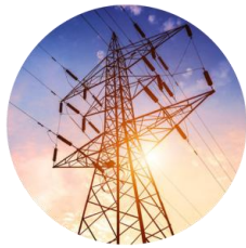
Power Transmission & Distribution
