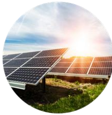
Solar EPC Projects
